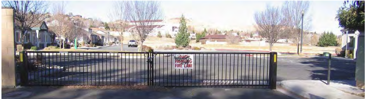
Existing Fence/Emergency Access/Pedestrian Access at Holman Way
